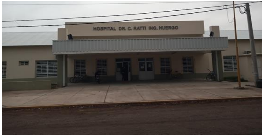
Hospital Ing. Huergo – Almacenamiento final RBP-RQP
